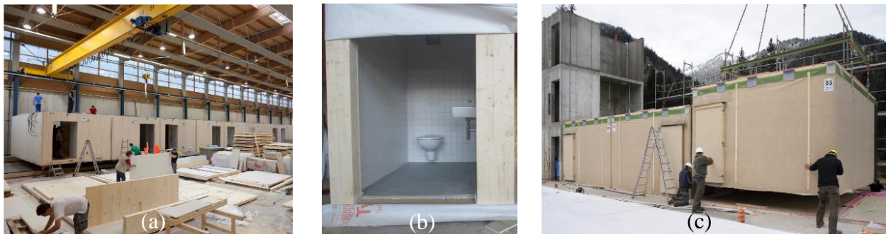
Figure 1. (a) Production facility of CLT room modules in Austria; (b) fully equipped bathroom inside a module; (c) module assembly at the construction site.
