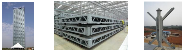
Figure 1. T30 hotel building. Figure 2. Main floor. Figure 3. Inclined-brace column.
