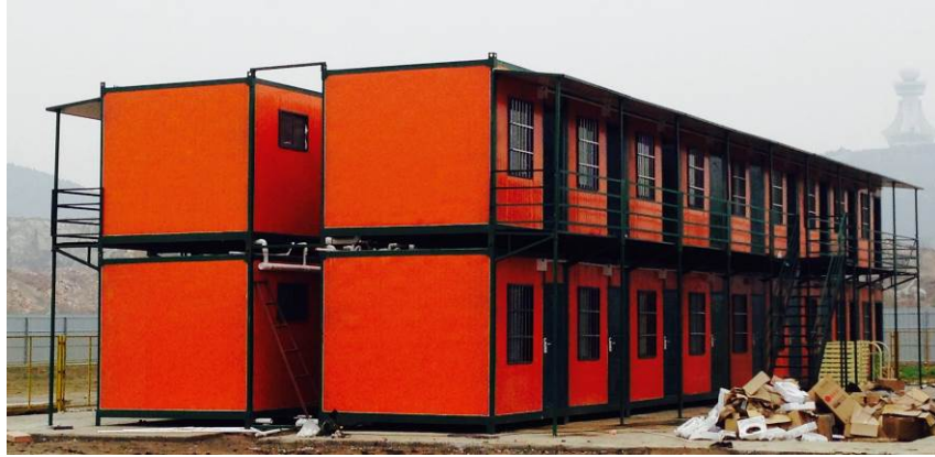
Figure 4. Double deck quarters on site (half finished)
