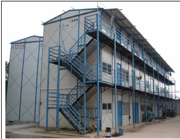
Figure 1. Temporary quarters for migrant construction on-site workers
