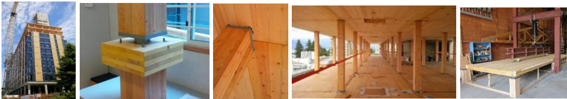
Figure 1. CLT slab-on-post structural system adopted for the UBC Brock Commons and monotonic tests conducted at FPInnovations ( courtesy of naturallywood and FPInnovations )
