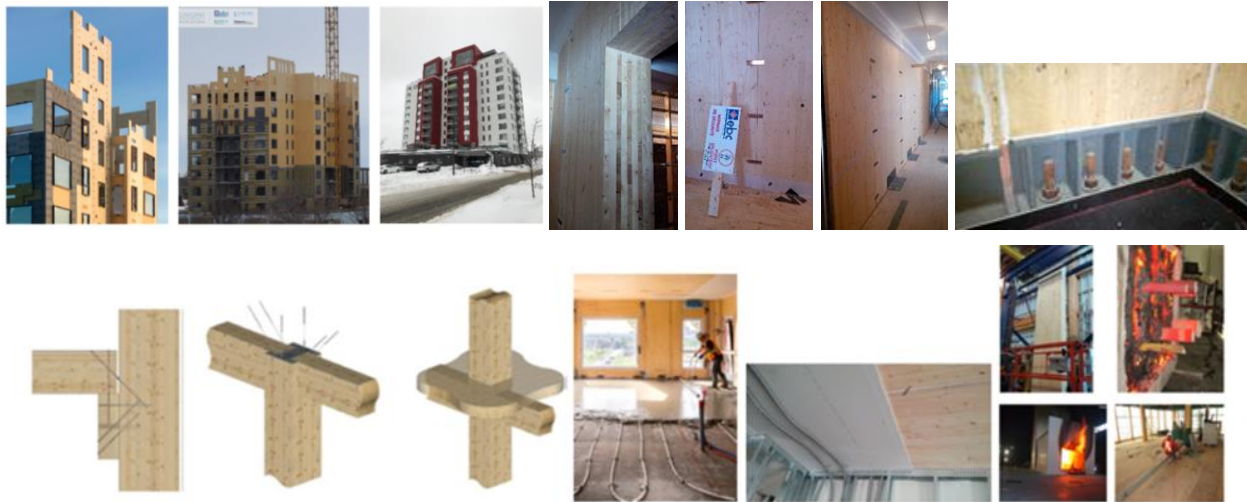
Figure 3. Quebec’s 13-storey building: details on CLT shearwalls, holddowns, connections and fire and structural testing (courtesy of Stéphane Groleau, Nordic Structures and FPInnovations).
